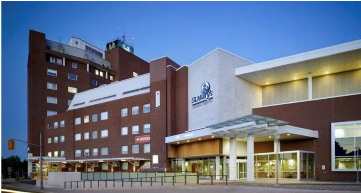
Picture 1. St. Mary’s General Hospital
